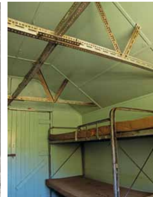
Interior of Back Ridge Hut showing original Dexion framing, 2004. PHOTO: SHAUN BARNETT/BLACK ROBIN PHOTOGRAPHY
